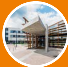
ZMK Hospital, Netherlands
